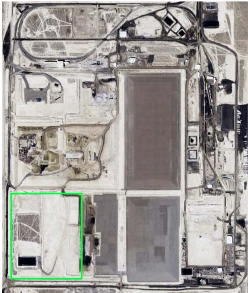
Figure 1. The Clive Facility, with the location of the Class A South embankment outlined in green. This orthophotograph is roughly 1 mile across, and north is up.
